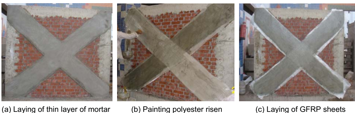
Fig. 4. Procedures of retrofitting walls by GFRP.
