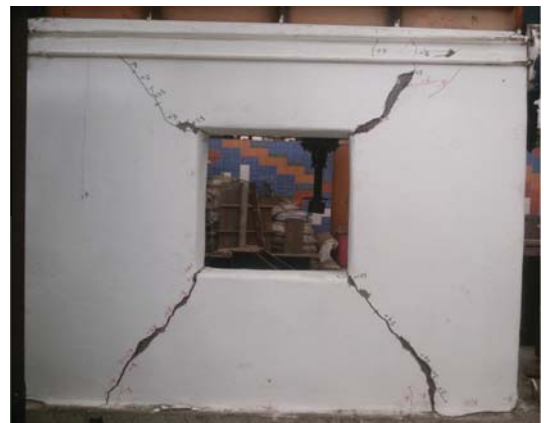
Fig. 17. Crack pattern for CLY-W-FERRO.
