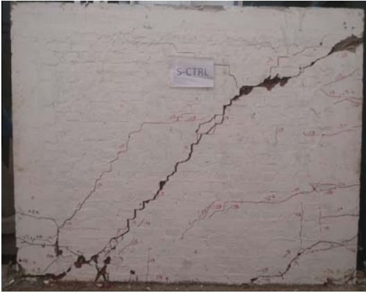
Fig. 10. Crack pattern for CLY-S-CTRL.
