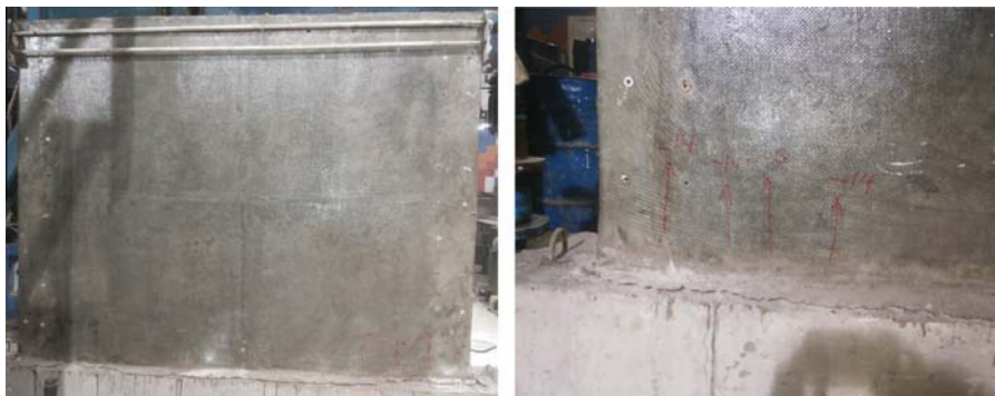
Fig. 15. Crack pattern for CLY-S-GFRP-F with enlarged rocking at connection.
