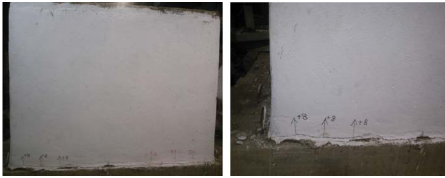
Fig. 14. Crack pattern for CLY-S-FERRO-F with enlarged rocking at connection.
