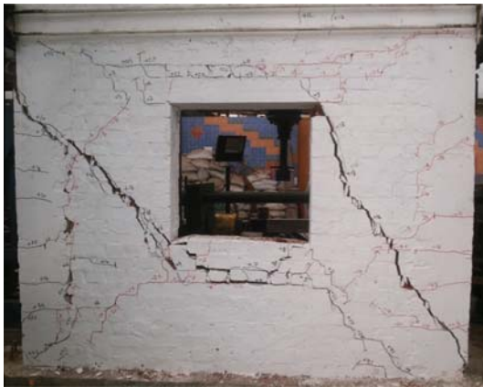
Fig. 16. Crack pattern for CLY-P-W.
