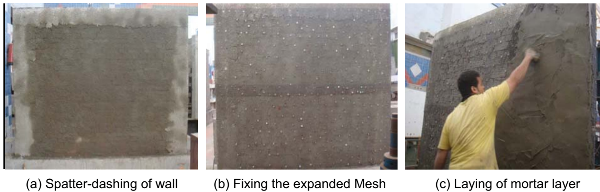
Fig. 3. Procedures of retrofitting walls by ferrocement.
