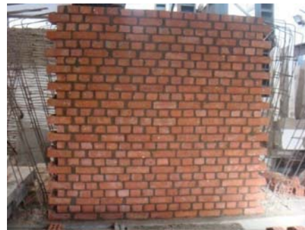
(b) Masonry wall construction
