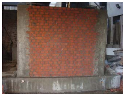
(c) Concrete casting of tie column
