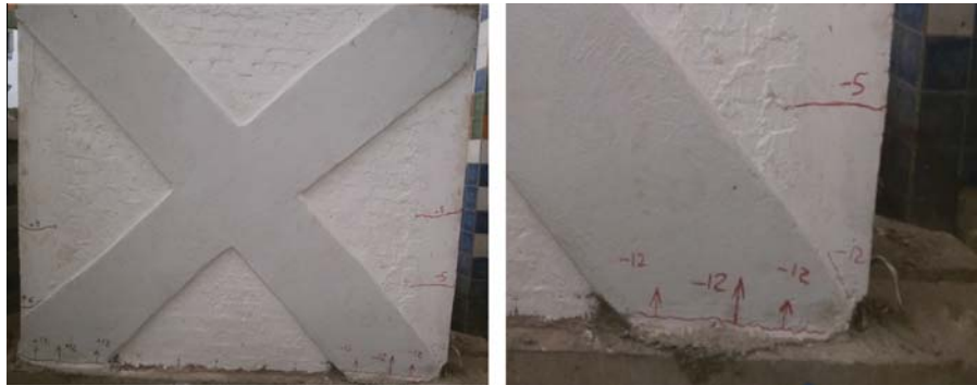
Fig. 12. Crack pattern for CLY-S-FERRO-X with rocking at connection.
