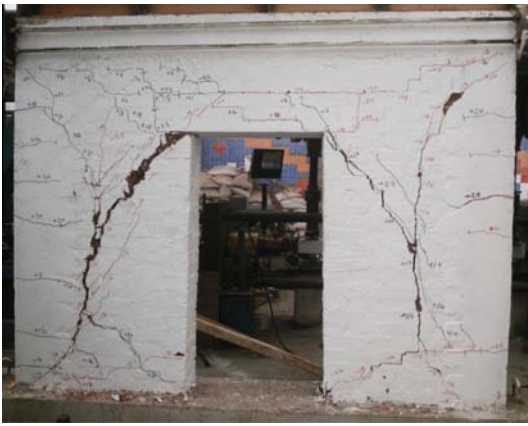
Fig. 18. Crack pattern for CLY-P-D.
